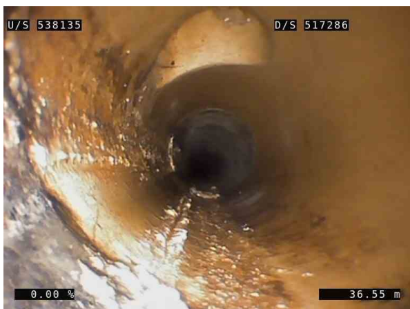
29, 00:05:18, 36.55m (9.79m) The lateral is open at 9 o'clock / 100mm
