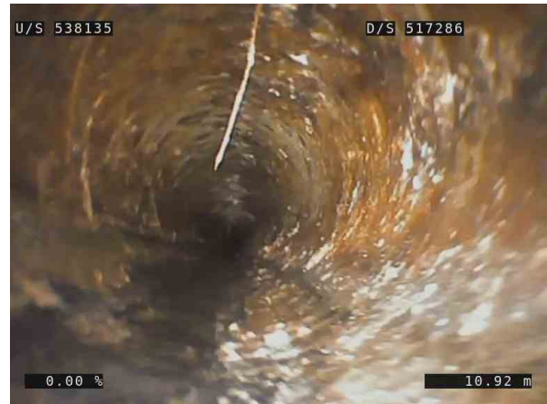
10, 00:01:41, 11.35m (34.99m) Fine roots, roots restrict flow by 10% or less of full flow from 10 o'clock to 12 o'clock
