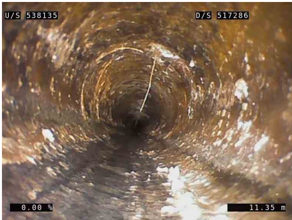
9, 00:01:41, 11.35m (34.99m) The sealing of the joint is faulty, large, clearly through the pipe wall from 10 o'clock to 12 o'clock / RIFS
