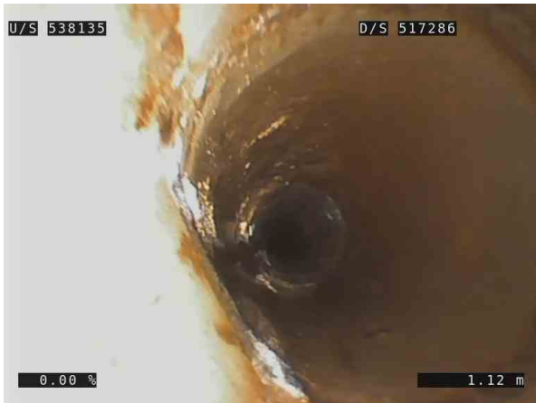
5, 00:00:46, 1.10m (45.24m) Obstruction permanent, reduction of up to 10% of the pipe diameter from 5 o'clock to 7 o'clock / Grout
