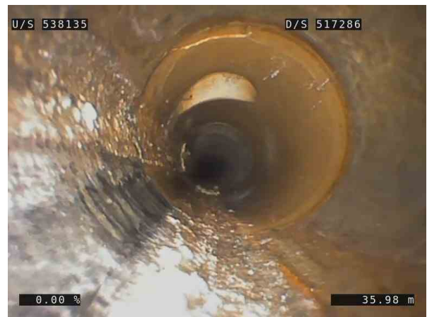
28, 00:05:09, 36.21m (10.13m) Joint faulty, medium cracking or spalling, probably through the pipe wall from 7 o'clock to 12 o'clock
