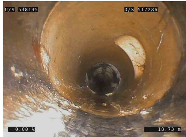
18, 00:03:08, 18.45m (27.89m) Fine roots, roots restrict flow by 10% or less of full flow from 2 o'clock to 5 o'clock
