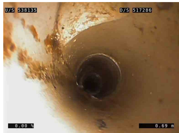
4, 00:00:44, 0.69m (45.65m) The lateral is open at 9 o'clock / 100mm
