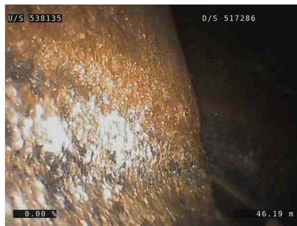
32, 00:07:15, 46.19m (0.15m) Debris silt, small, clear diameter reduced by less than 10%, end / Gravel stones
