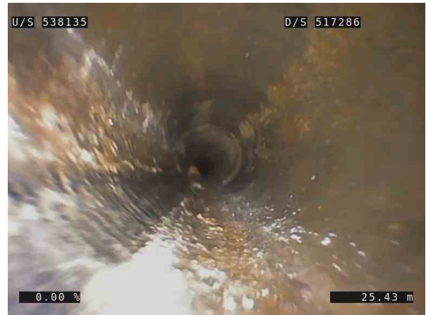
22, 00:03:48, 25.43m (20.91m) Debris greasy, small, clear diameter is reduced by less than 10% from 10 o'clock to 2 o'clock, end / Pipe roof
