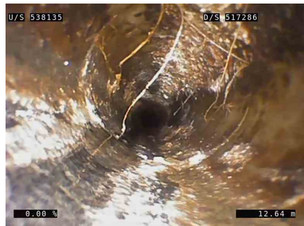
12, 00:01:58, 12.64m (33.70m) The sealing of the joint is faulty, large, clearly through the pipe wall from 9 o'clock to 2 o'clock / RIFS
