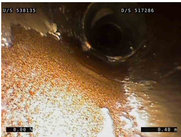
3, 00:00:41, 0.40m (45.94m) Debris greasy, small, clear diameter is reduced by less than 10% from 12 o'clock to 12 o'clock, start / Fat - Grease
