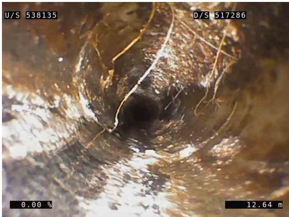
13, 00:01:58, 12.64m (33.70m) Fine roots, roots restrict flow by 10% or less of full flow from 9 o'clock to 2 o'clock
