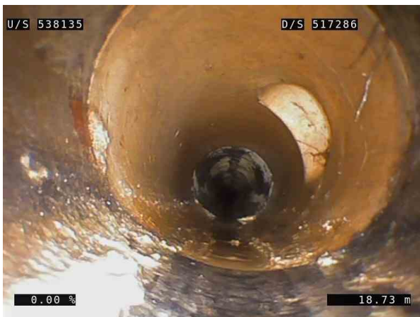
19, 00:03:07, 18.73m (27.61m) The lateral is open at 2 o'clock / 100mm
