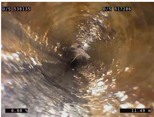
11, 00:01:53, 11.49m (34.85m) Debris greasy, small, clear diameter is reduced by less than 10% from 10 o'clock to 2 o'clock, start / Pipe roof
