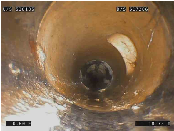
17, 00:03:08, 18.45m (27.89m) The sealing of the joint is faulty, large, clearly through the pipe wall from 2 o'clock to 5 o'clock / RIFS
