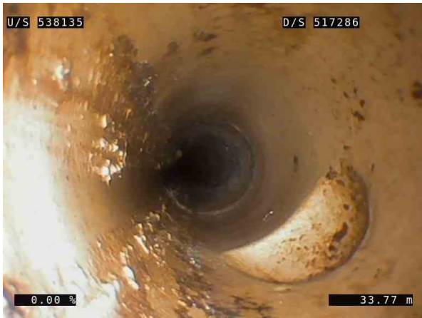
25, 00:04:44, 33.77m (12.57m) The lateral is open at 2 o'clock / 100mm
