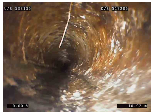
8, 00:01:41, 11.35m (34.99m) The sealing of the joint is faulty, large, clearly through the pipe wall from 10 o'clock to 12 o'clock / RIFS
