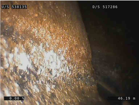
33, 00:07:15, 46.19m (0.15m) Debris greasy, small, clear diameter is reduced by less than 10% from 4 o'clock to 8 o'clock, end / Pipe walls
