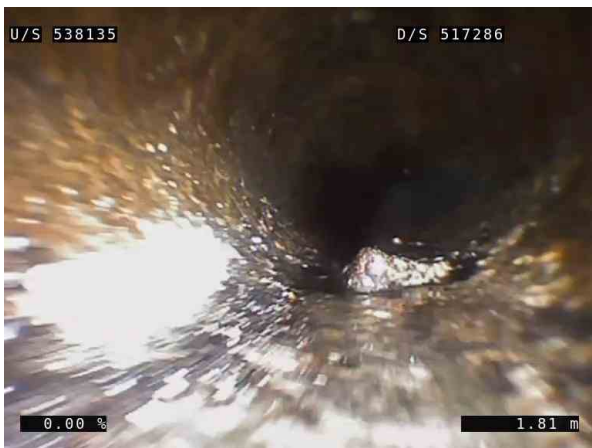
7, 00:00:49, 1.81m (44.53m) Debris silt, small, clear diameter reduced by less than 10%, start / Gravel stones
