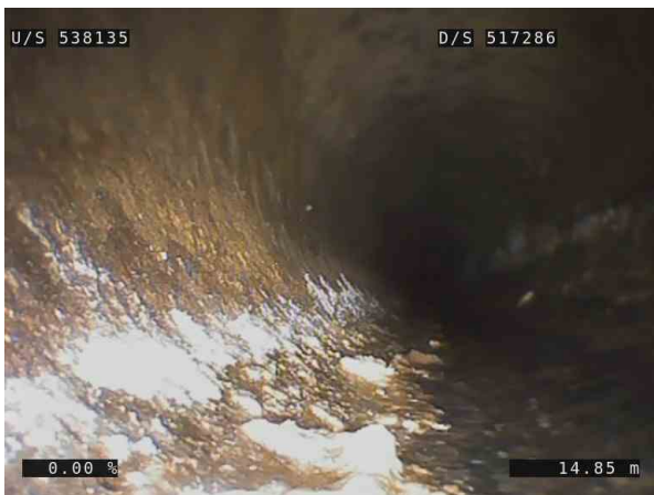
15, 00:02:30, 14.85m (31.49m) Fine roots, roots restrict flow by 10% or less of full flow from 9 o'clock to 2 o'clock
