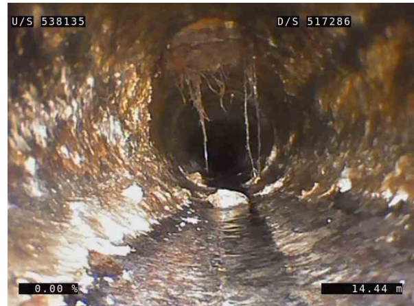
14, 00:02:22, 14.44m (31.90m) Lateral sealing faulty, evidence exist that the connection between the lateral and the main pipe is leaking at 12 o'clock / 100mm. Roots via seal
